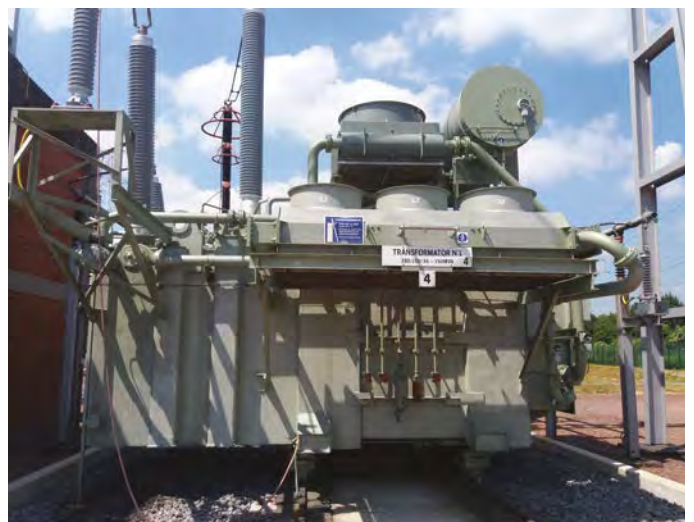
Full retrofit of 400 kV transformer
